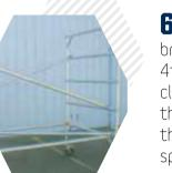
**6.** Attach 2 diagonal braces (blue) to 2nd & 4th rung of frame with claw facing down. Level the unit by turning the lever on the wheel spindle.
