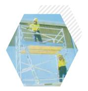
**15.** Outriggers must be fitted to all mobile scaffolds when working platform height is 3 times the minimum width of base unit.
