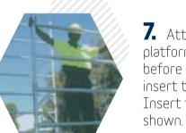
7. Attach the fixed platform to the 3rd rung before attempting to insert the extensions. Insert frames (2) as
