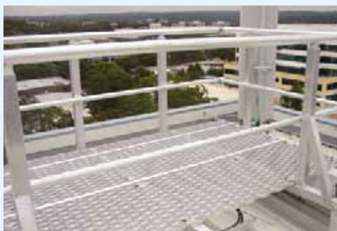
TYPICAL APPLICATION OF ROOF WALKWAY WITH HANDRAIL
