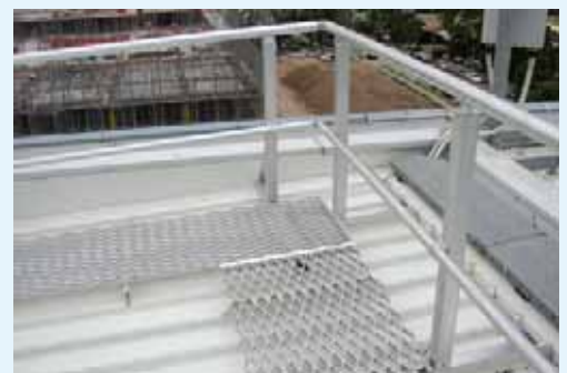
TYPICAL APPLICATION OF ROOF WALKWAY WITH HANDRAIL
