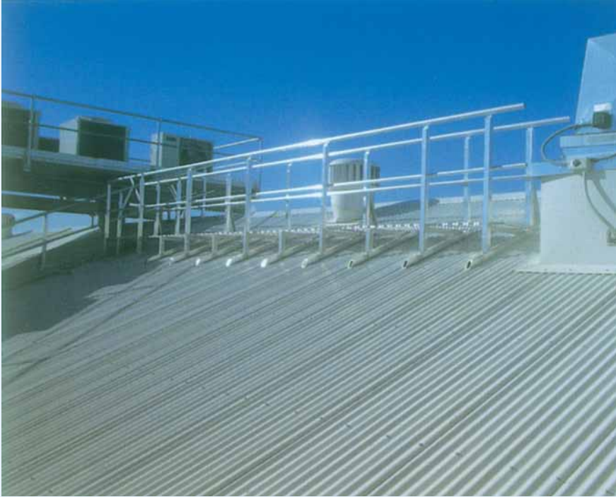
Typical installation showing handrail posts 'vertical'
